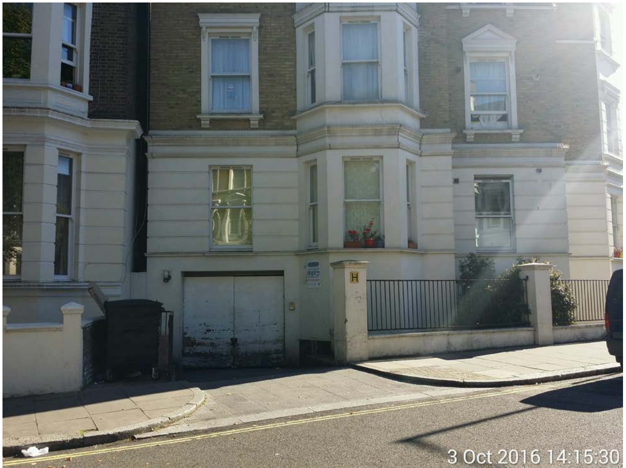
Photo to show garage doors of 1 Elgin Avenue (accessed from Walterton Road)
